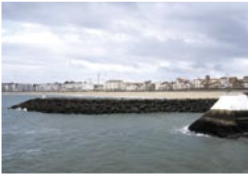
3. Manmade structure (ESI 2)
